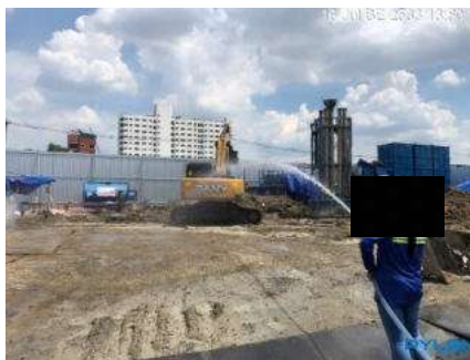
11. Spraying water to reduce dust.
